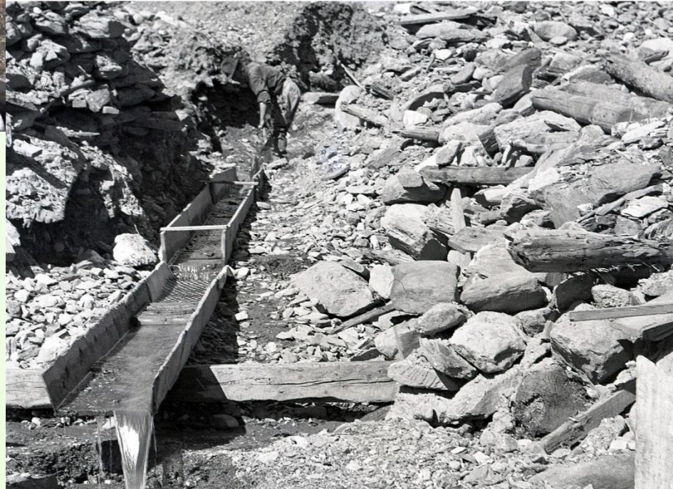
Long sluice trough
